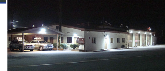
U. S. Army Garrison Humphreys, Republic of Korea: LEDtronics LED Wall-Paks illuminate the four bay doors (top) at the camp's fire station, while the rest of the building is lit with standard 250W HPS (amber glow). (Above) The building now updated with a full complement of LEDtronics WWL20 Wall-Pack units.
